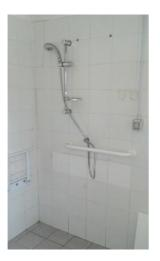
The shower room that doubles as a dressing room is separated from the toilet room SEBACH and can be reached via the small step of 0.5 cm knockers. The useful width of the front door is> 80 cm. The shower is at floor level, open-ended and it has a folding seat. It 'a support handle and from a sitting position you can reach the faucet. To the side is an electric bell to unreachable from the ground button. The internal dimensions are: width 166 cm and 236 cm depth.
